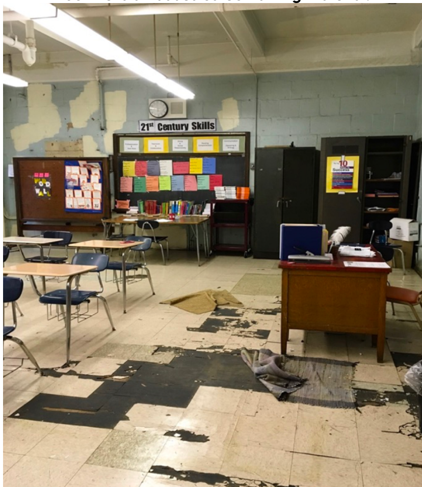
Photo 8—High School— Teacher described the conditions as existing for several months. The floor tile is an asbestos-containing material.
