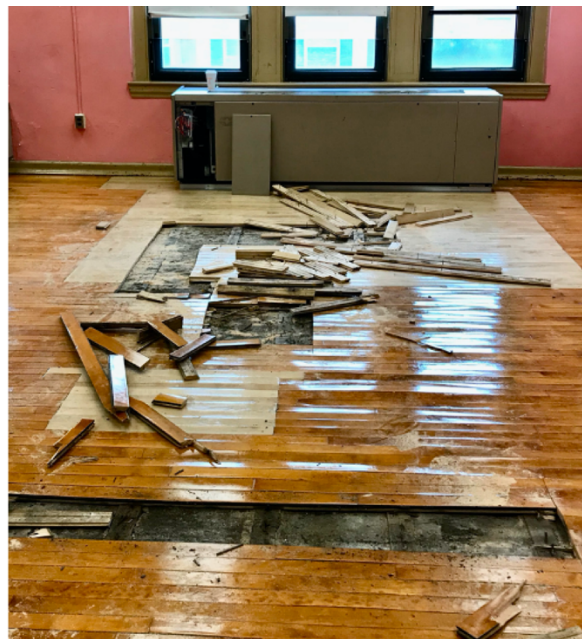
Photo 7 – Elem. Classroom — Repeat flooding from malfunctioning classroom unit ventilator resulting in extensive damage and mold growth to newly installed flooring — the original flooring was replaced for the same reason just a few weeks earlier. An example of what happens if the “root causes” are not addressed and also issues related to inadequate governance, oversight, and management
