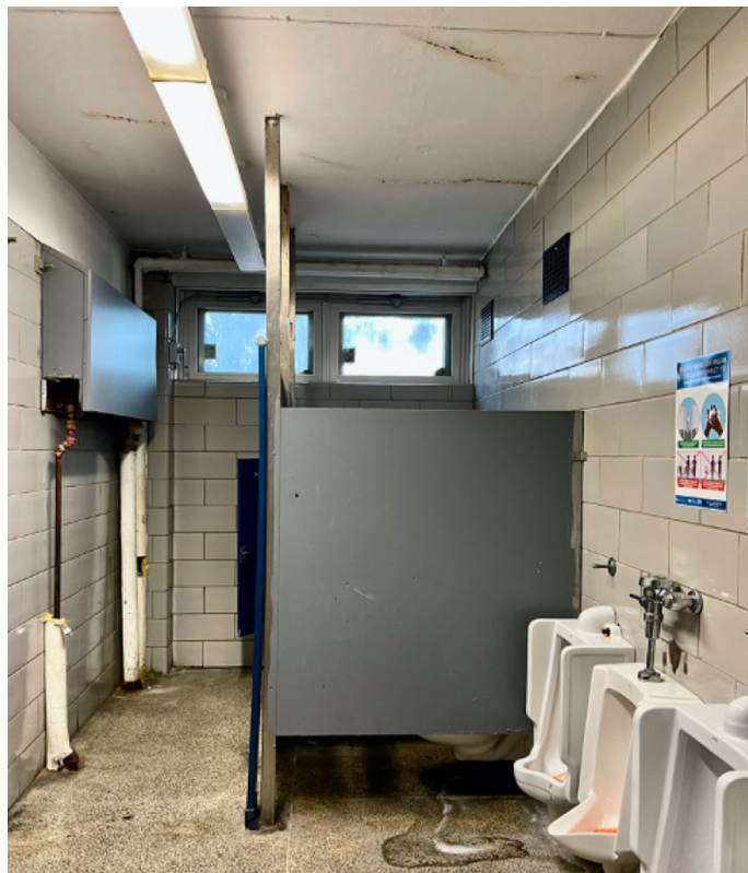
Photo 10 – Elem. Boys Bathroom— Filthy conditions, leaks on floor and ceiling deteriorated/damaged and missing insulation on piping presenting a burn hazard from very hot heating pipes.
