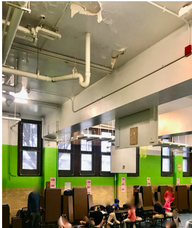
Photo 3 – Occupied Gym/Lunchroom— Kids sitting and eating underneath severely damaged lead painted ceiling
